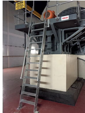
Companionway / ships ladder to existing platform
